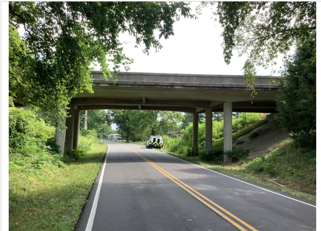
Underclearance looking back on underpass route
