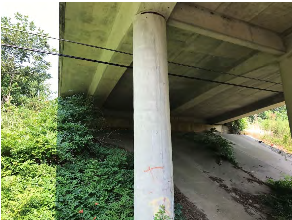
Underside of bridge looking west (featuring utilities)
