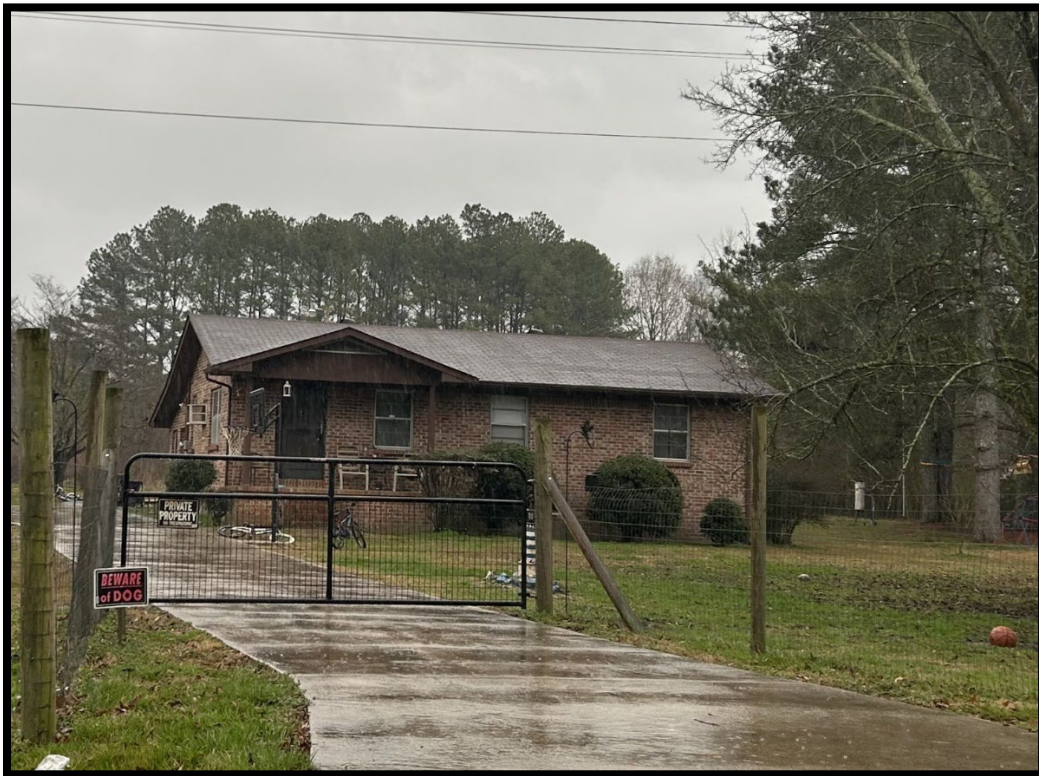
Figure 6: Front (western) façade of HS-1.
