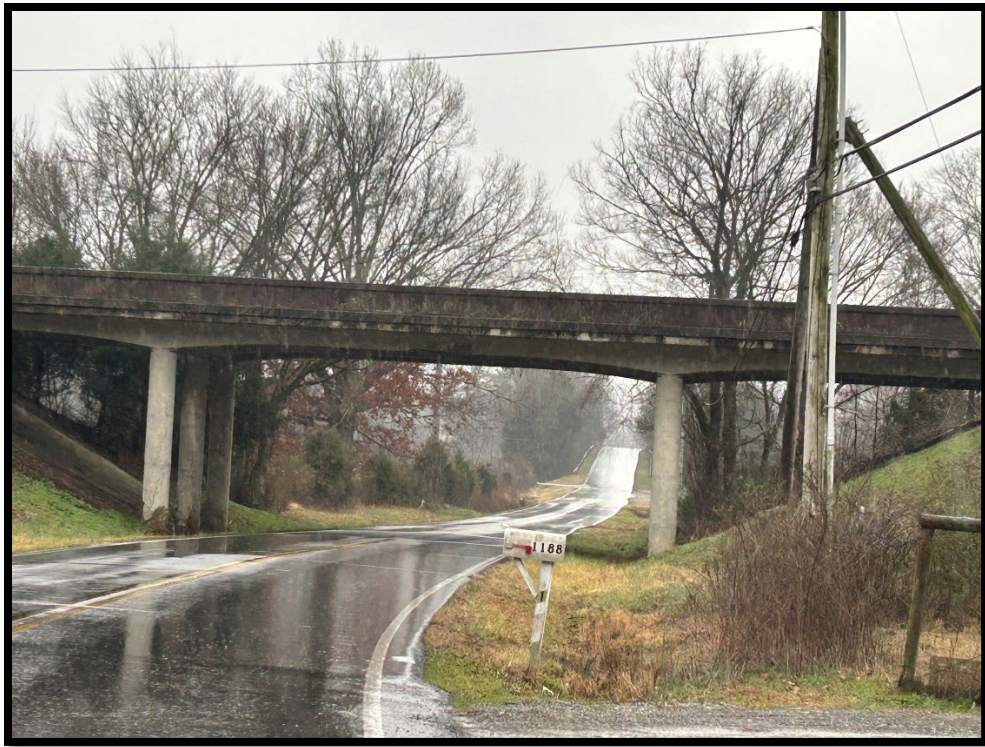
Figure 13: I-24 bridge looking south.
