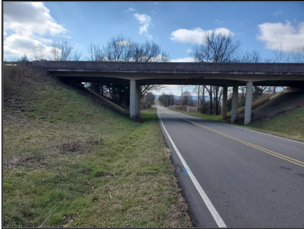
Figure 4. Bridge over Shellmound Road, facing south.
