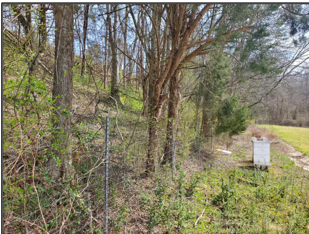
Figure 8. Berm to the south of I-24, facing northeast.
