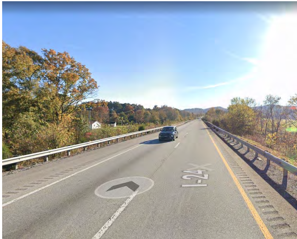
Western Approach Looking East
