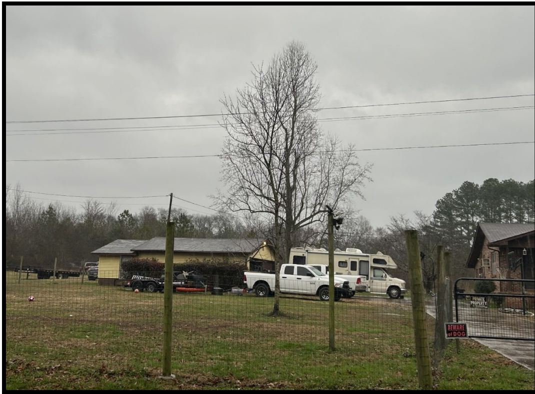
Figure 8: Outbuilding surveyed with HS-1.
