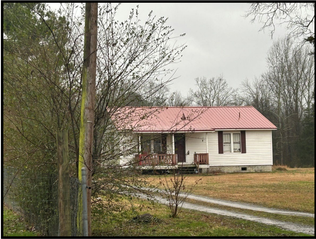
Figure 10: Side view of HS-2, looking southeast.
