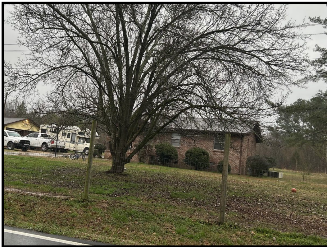
Figure 7: Side view of HS-1, looking east/northeast.
