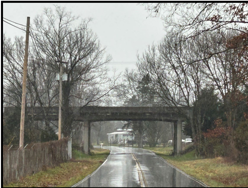
Figure 13: I-24 bridge looking north.
